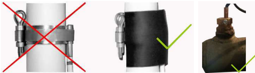
Pic. No. 8 – Thermal sensor installation
