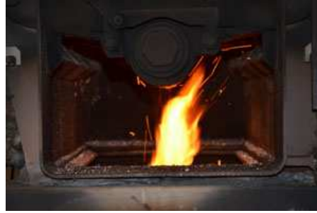
Pic. No. 14 Poor flame shape
