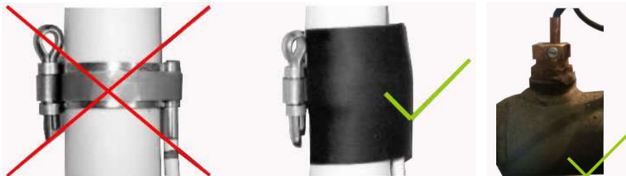
Pic. No. 8 – Thermal sensor installation
