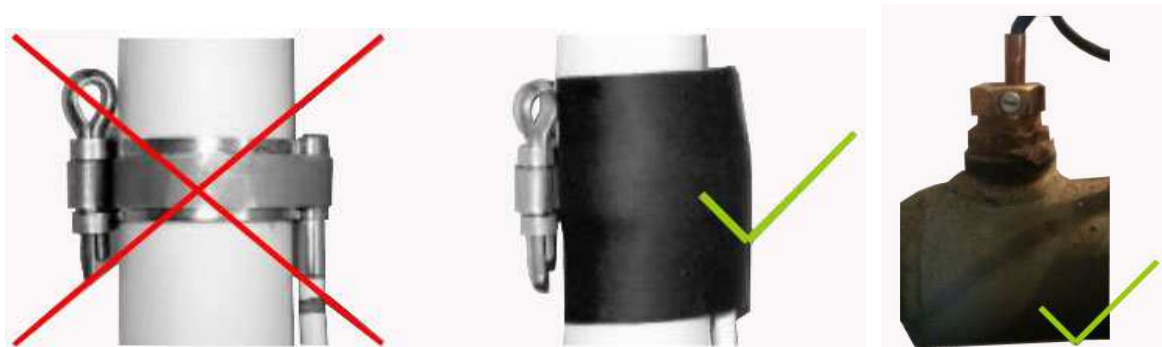
Image 4 – Thermal sensor installation
